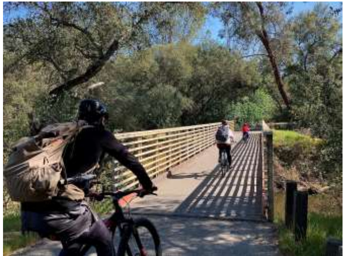
Willow Creek Bridge
