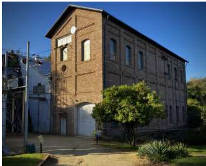
Folsom Powerhouse SHP, Main Powerhouse
